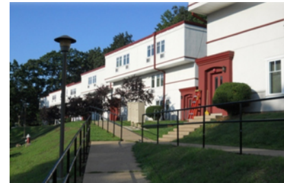
Hawk Crossings Dormitory Complex, Montclair State University
